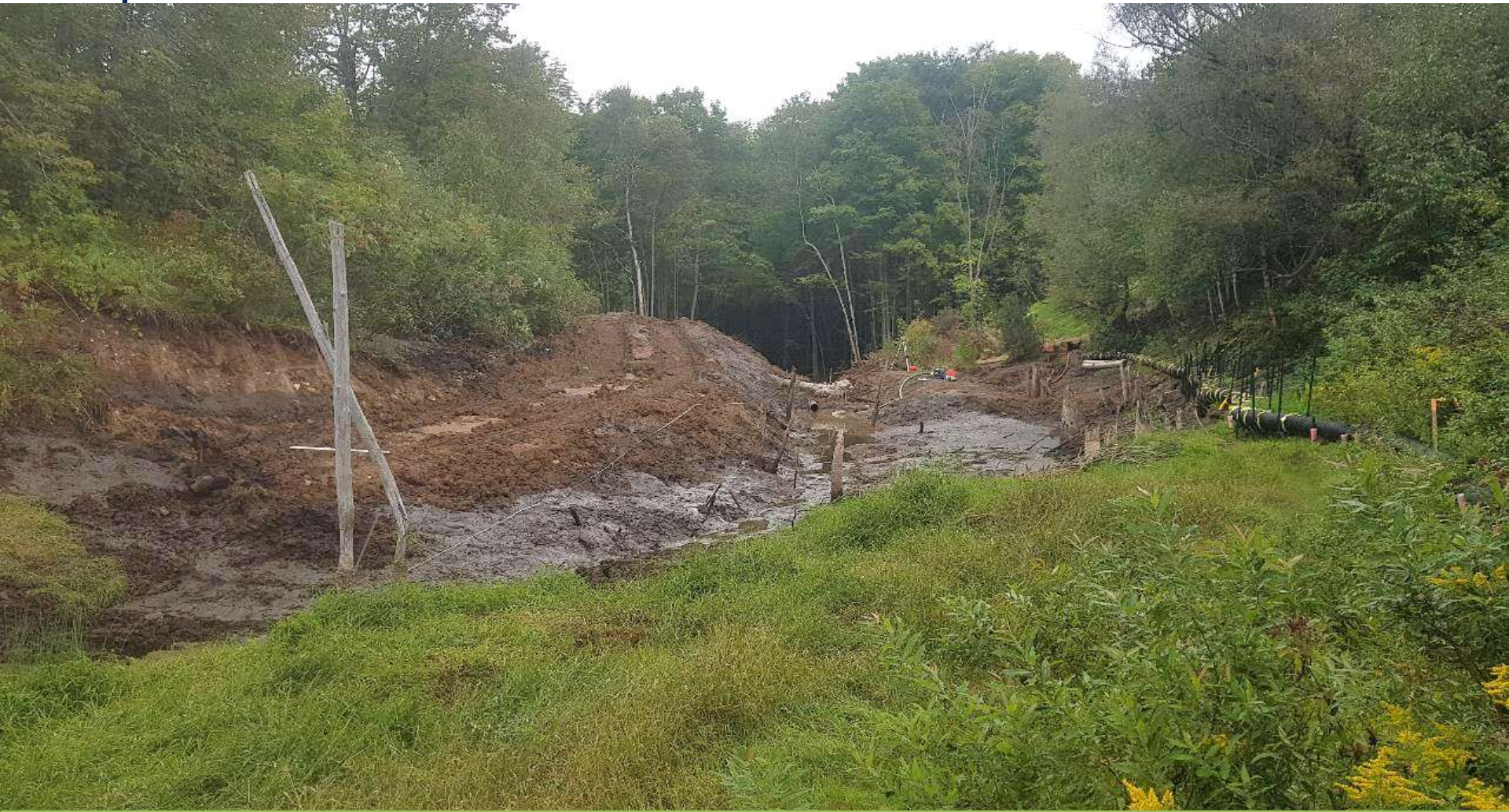
Berm Excavation and Sediment Removal Sept 2020
