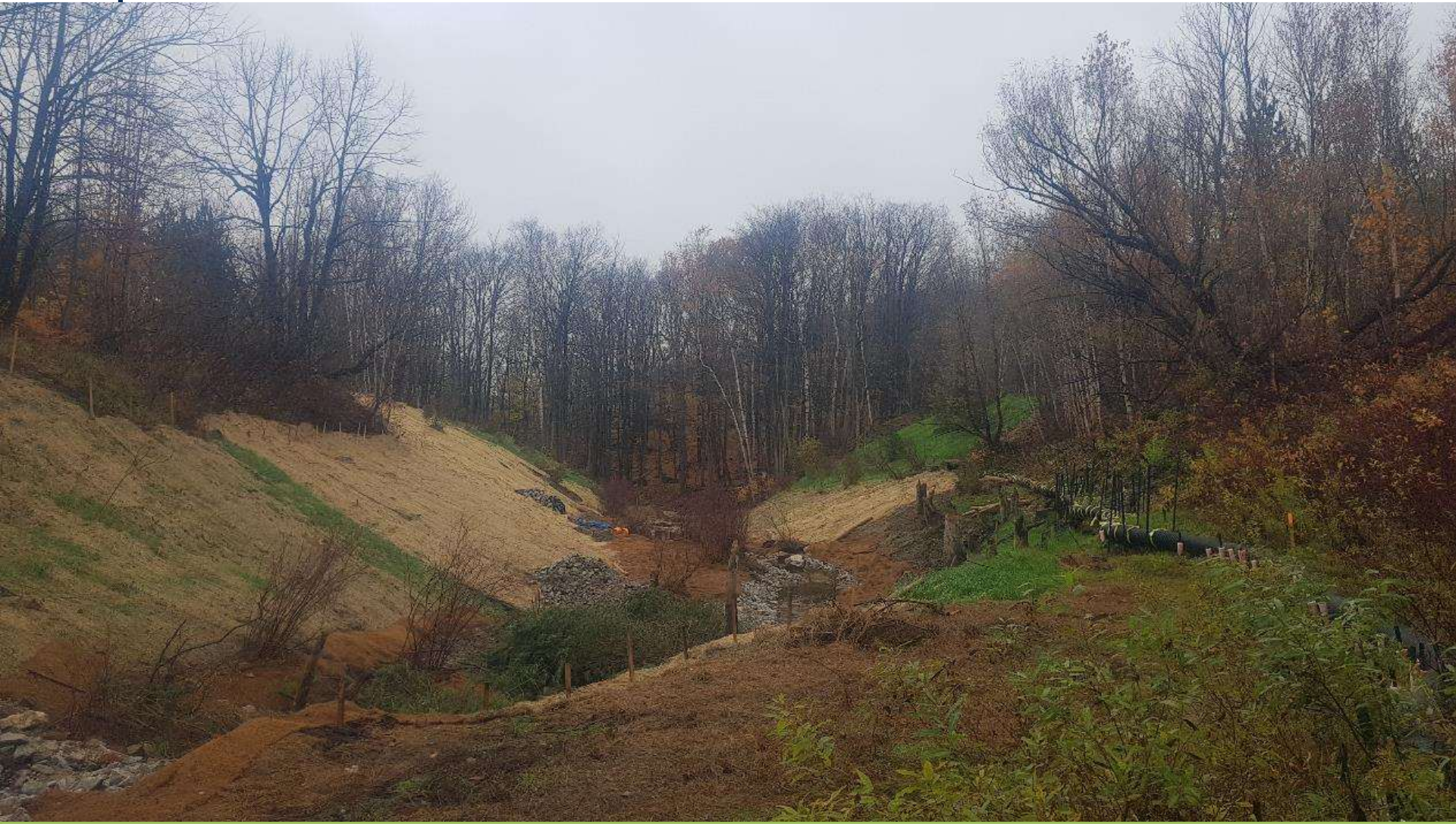
After Dam Removal and Channel Construction Oct 2020
