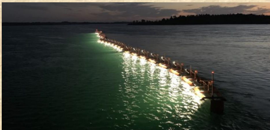
Figure 1: Photo of the light array outside Iroquois Water Control Dam, September 2022
