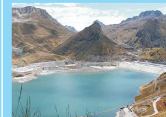
Image 6. Antamina mine impoundment.
