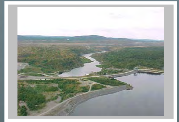
Steephill Falls Dam and Magpie River looking downstream.
