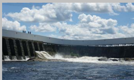
Photo left: Hydro dam at International Falls, MN. Photo courtesy of Bill Gardner
