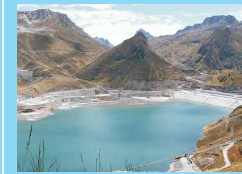
Image 6. Antamina mine impoundment.
